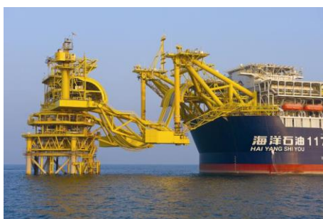
Peng Bo FPSO in Bohai Bay, China
